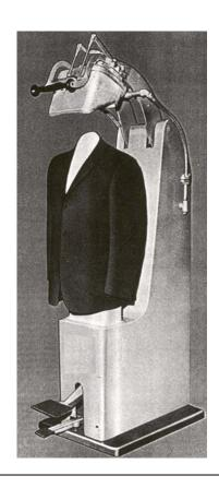
Korrect Kollar is designed to conform to the human contour. Thus collars pressed with this machine hug the neck gracefully and remain 'just so'.
